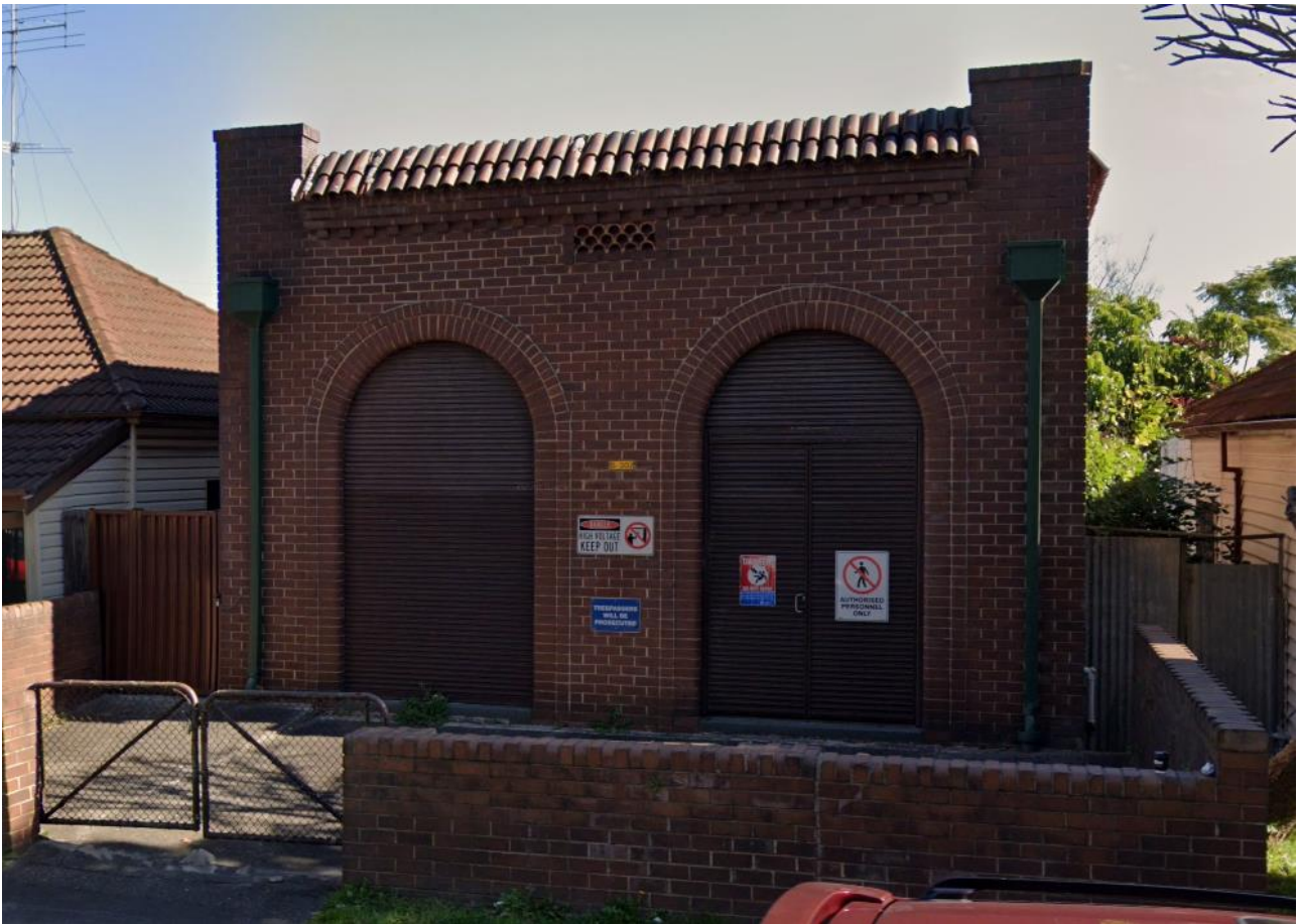
Figure 10 Sub-Station, 40A George Street, North Strathfield.
