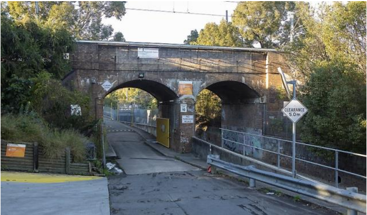
Figure 7 Railway Viaduct over Powell Creek (view south).
