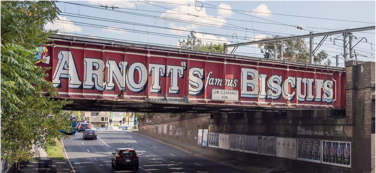
Figure 6 Arnott's advertisement on the railway bridge crossing Parramatta Road.
